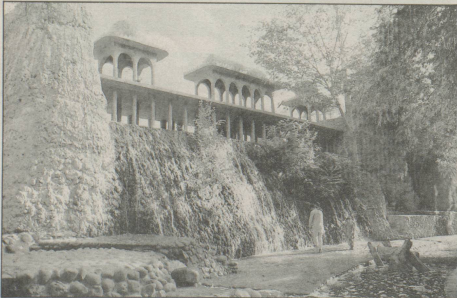
GRAND PALACE COMPLEX (New Extension): Summer pavillion of the Grand Palace has a trough that runs along its entire length. This is used as a water cascade. Structure atop the terrace is reminiscent of baradaris which were so frequently seen in Mughal and Rajput palaces.
